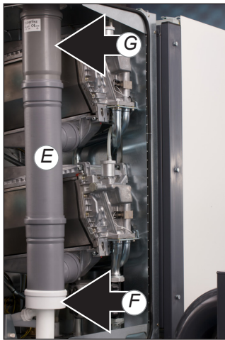
Removing flue pipe figure 13.3.b
