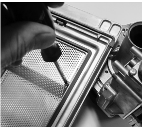
Removing gas air dividing plate
